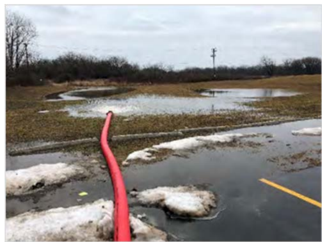
Figure 5.01-2 Pumping from 151st Street to Central Park Elementary School Detention Site (Jolly Homes CDBG Grant Application)
