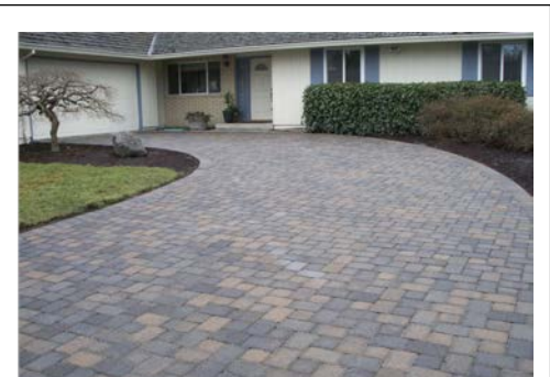
Figure 6.06-2 Pervious Driveway Pavers
