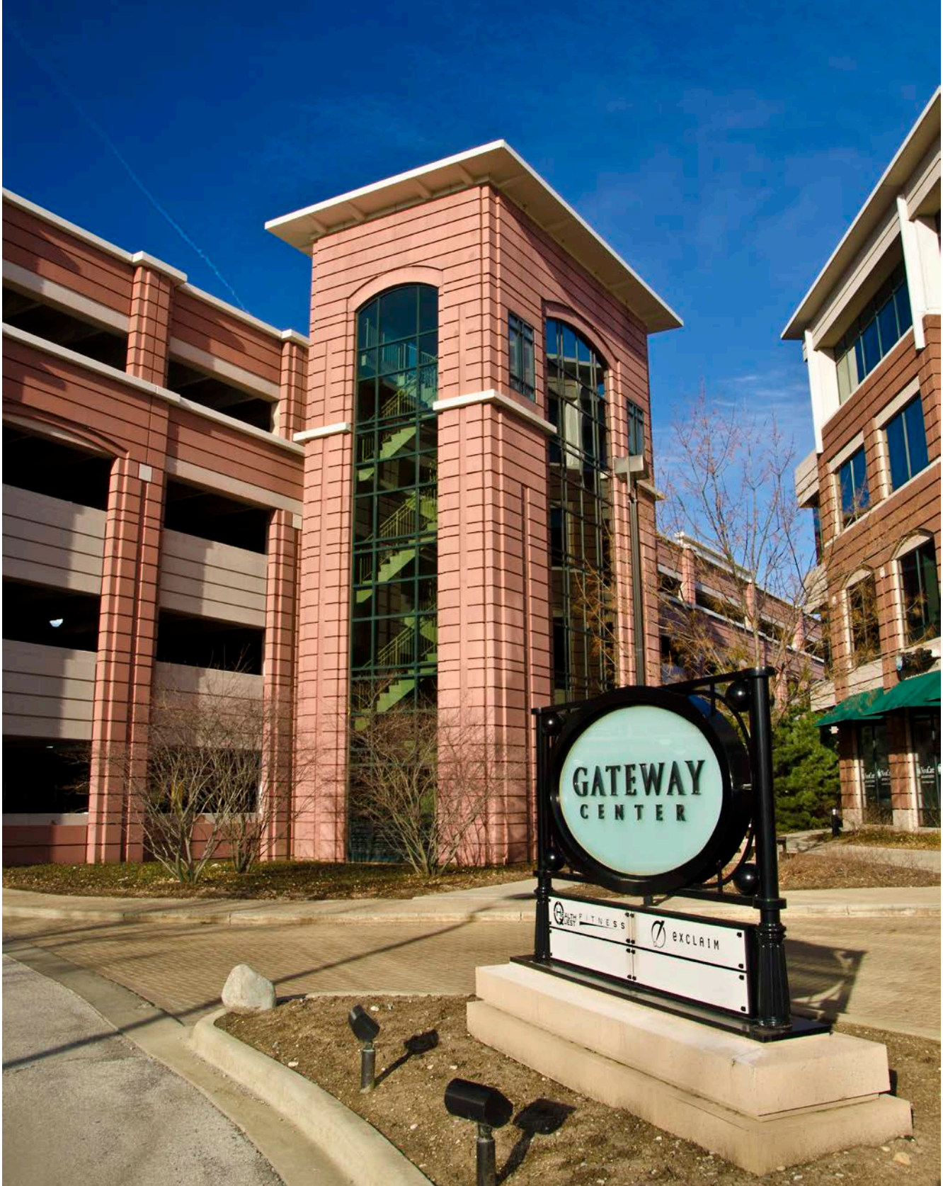
Palatine's Gateway Center is a four-story mixed-use parking deck with street level retail and office space on the upper floors adjacent to the Palatine Metra Station. Photo by Jim Watkins: http://www.flickr.com/photos/jim_watkins/
