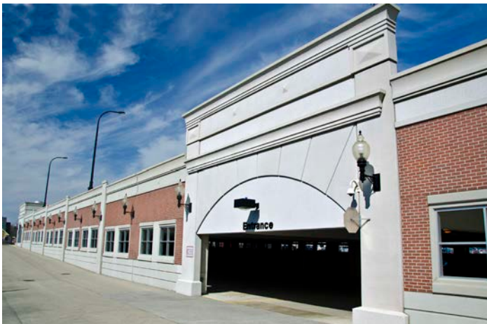
Geneva's municipal parking garage was engineered to accept a third level as additional funding became available and extra spaces were warranted. Photo by Jim Watkins: http://www.flickr.com/photos/jim_watkins/
