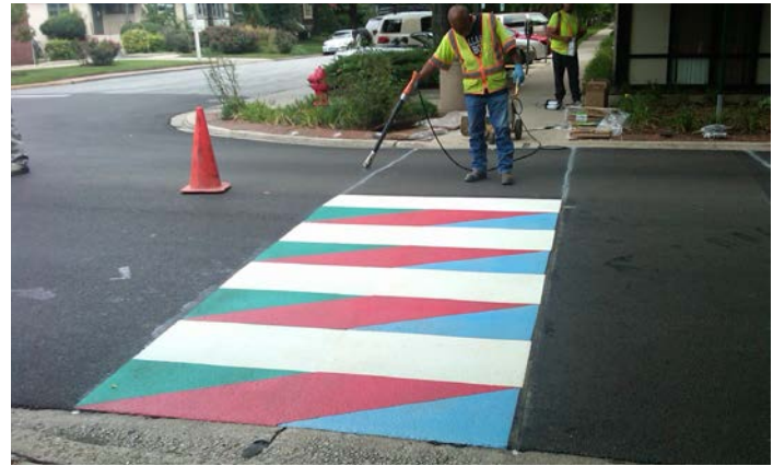
Enhancing crosswalks to promote pedestrian safety in Oak Park.
