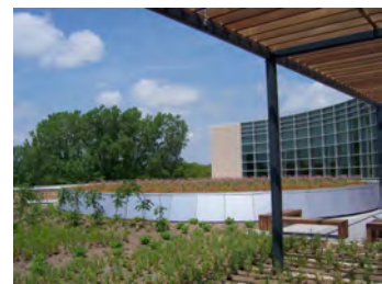
Green roofs on all new development buildings: Green roofs reduce heat island effect
