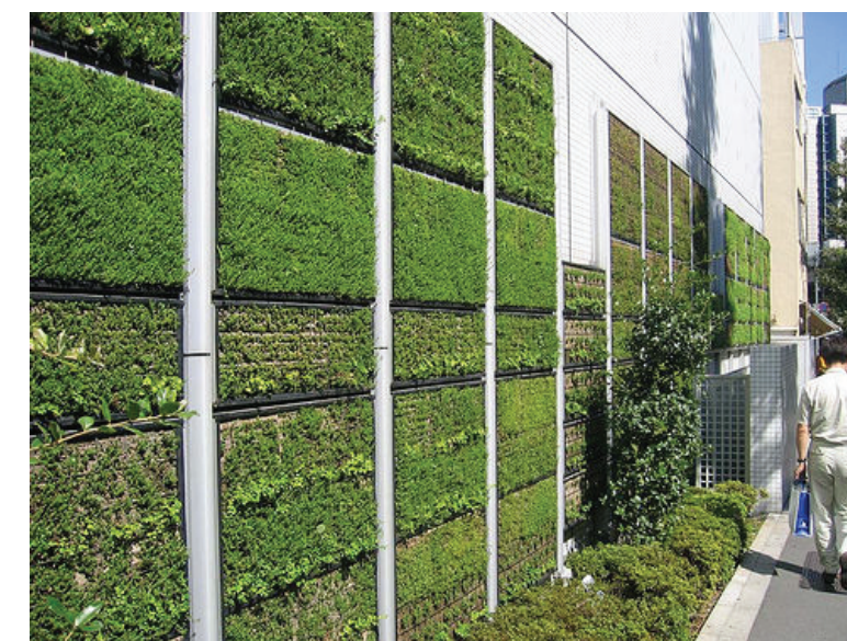
Vertical Green Wall
