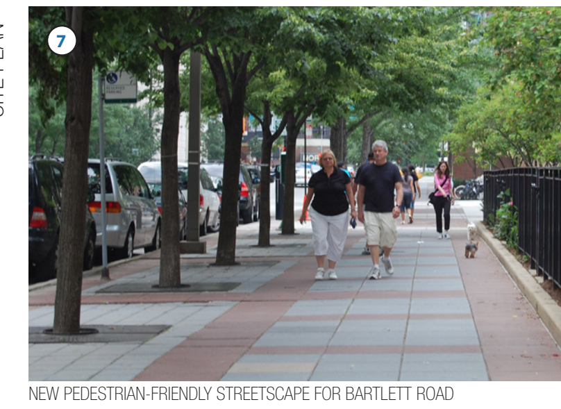
NEW PEDESTRIAN-FRIENDLY STREETScape FOR BARTLETT ROAD
