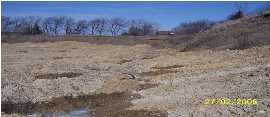
Pre-project conditions indicate 20-foot tall north and east boundary slopes contained erosion. Substantial deposits of eroding soil stockpiles were located along the disturbed area (photo by Sue Harney, Dundee Township).
