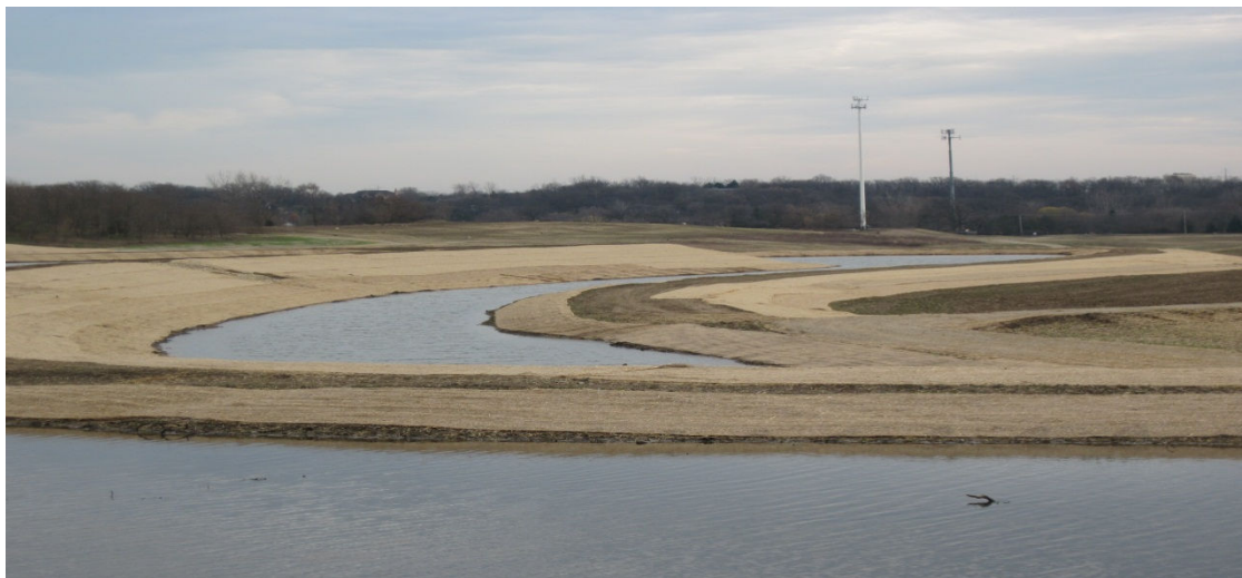
Post-Project conditions included conversion of eroding slopes into 4,000 linear feet of graded Terraced Swales. (photo by Sue Harney, Dundee Township).
