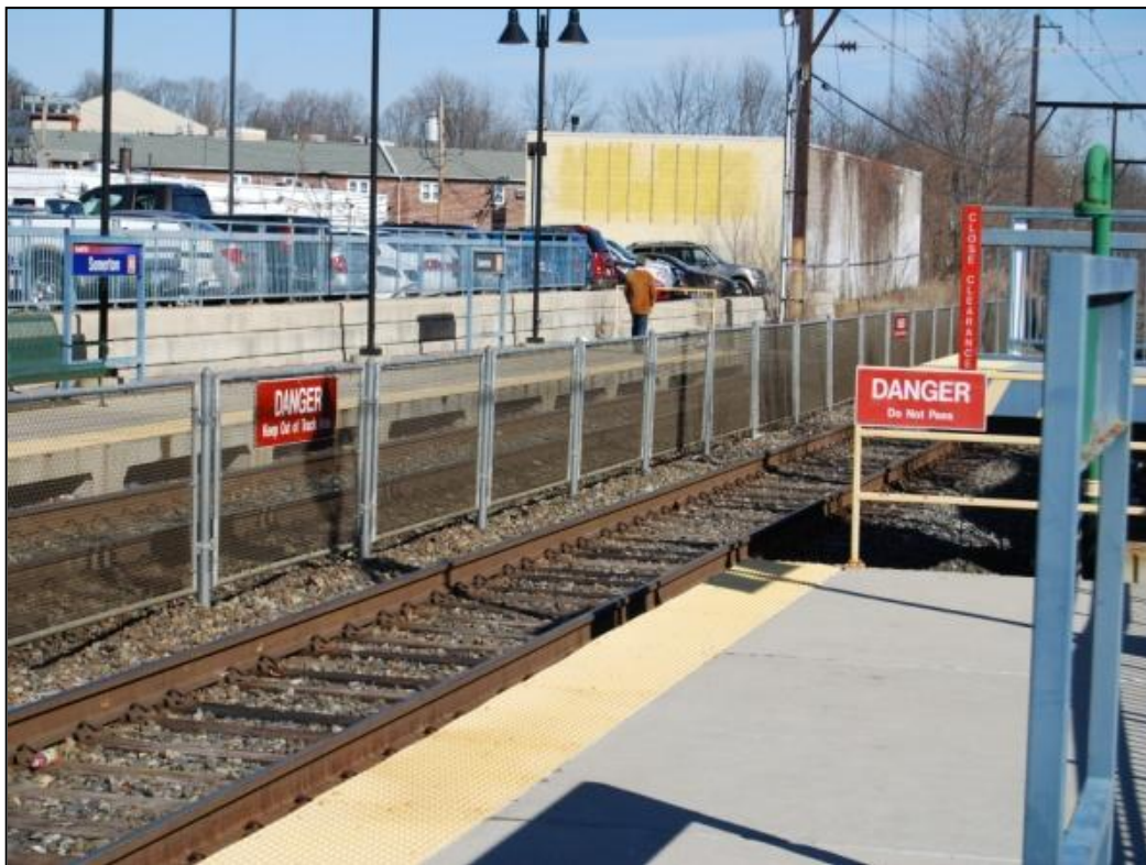
Figure 14: Example of station signing clearly indicating areas from which pedestrians are prohibited.
