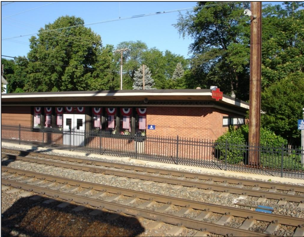
Figure 15: Example of platform edge fencing.
