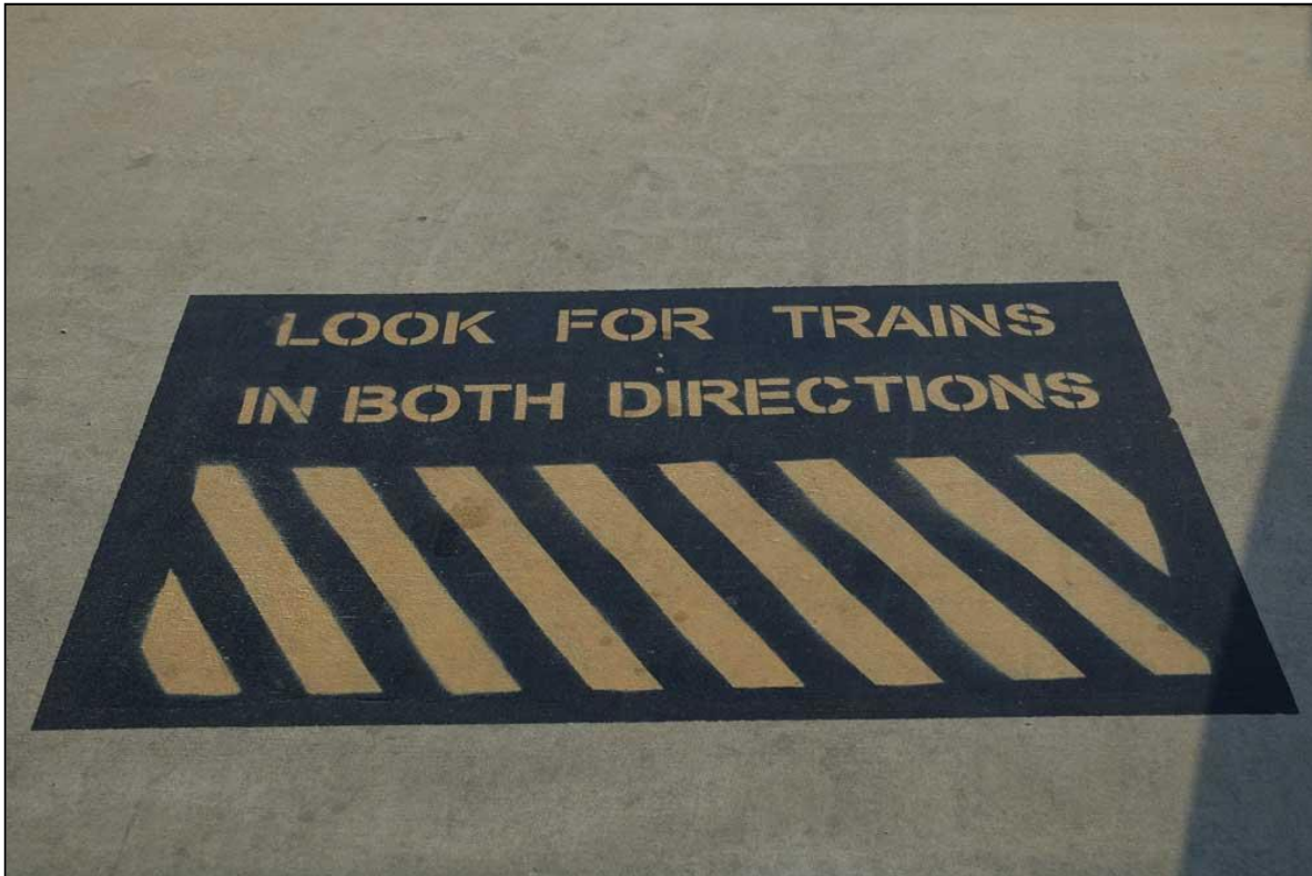
Figure 9: Example of a clear, concise warning message communicated by this pavement marking.
