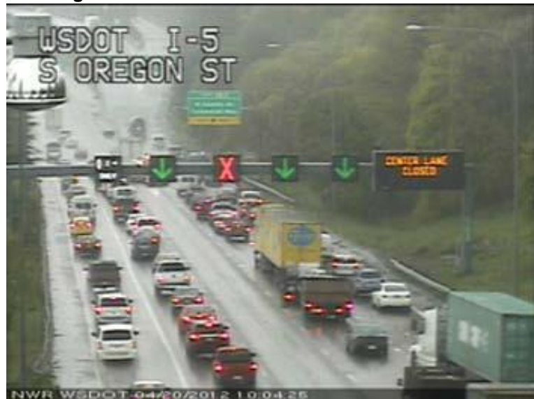
Figure 3. Example of active traffic management from Washington State
