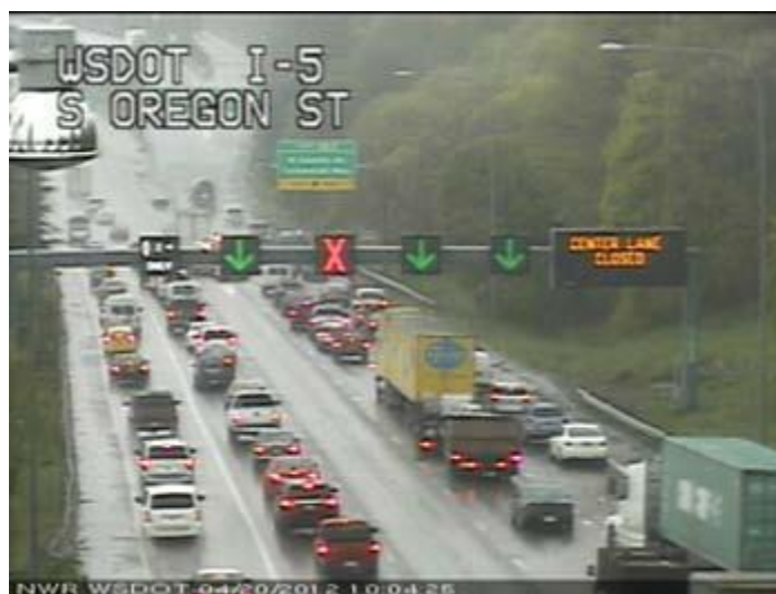
Figure 3. Example of active traffic management from Washington State
