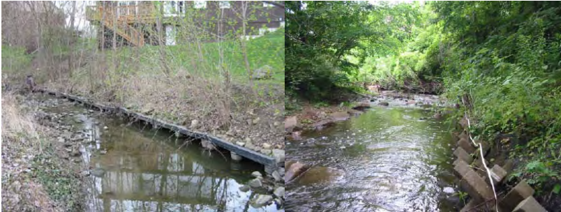
Figure 6-3. Left: Successful stabilization in Glencrest using lunkers. Right: Successful stabilization in Lockport using a-jacks.
