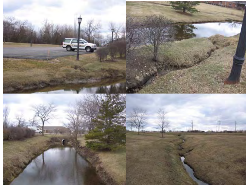
Figure 4-3. Above: Runoff from South Barrington Village Hall parking lot entering Poplar Creek. Below left: Erosion and sloughing behind Village Hall. Below right: Ditch from culvert under Barrington Rd in need of vegetative buffer.
