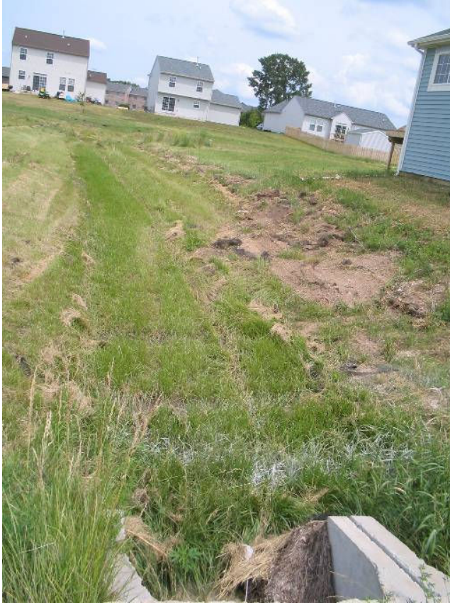
Figure 5-9: Facing east from end of 6 th Street, newly constructed swale.
