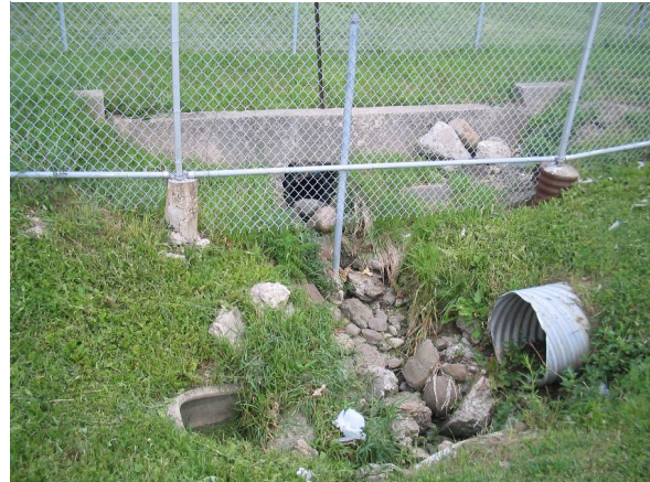
Figure 5-12: Facing east from Route 14, convergence of four drainage pipes next to high school.
