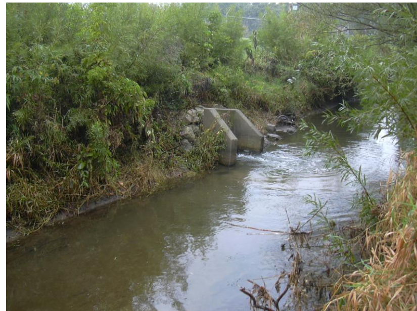
Figure 4-2. New Lenox WWTP #2 outfall
