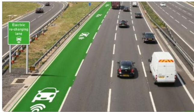
Figure 19. Electric Recharging Lane
