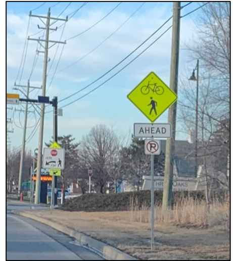
Figure 3-20. Advanced Pedestrian/Bicyclist Warning Signage
