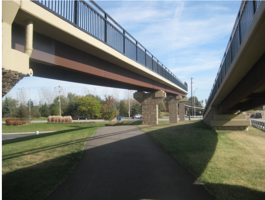
Figure 2.6: Pedestrian bridge over Randall Road, St. Charles
