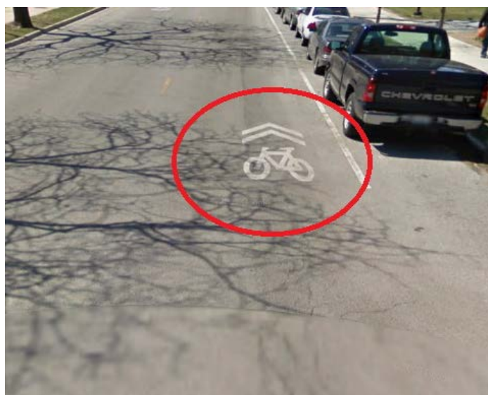
Figure 2.3: 33 rd Street shared lane identifier
