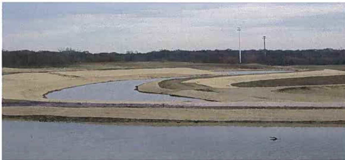
Post-Project conditions included conversion of eroding slopes into 4,000 linear feet of graded Terraced Swales. (photo by Sue Harney, Dundee Township).
