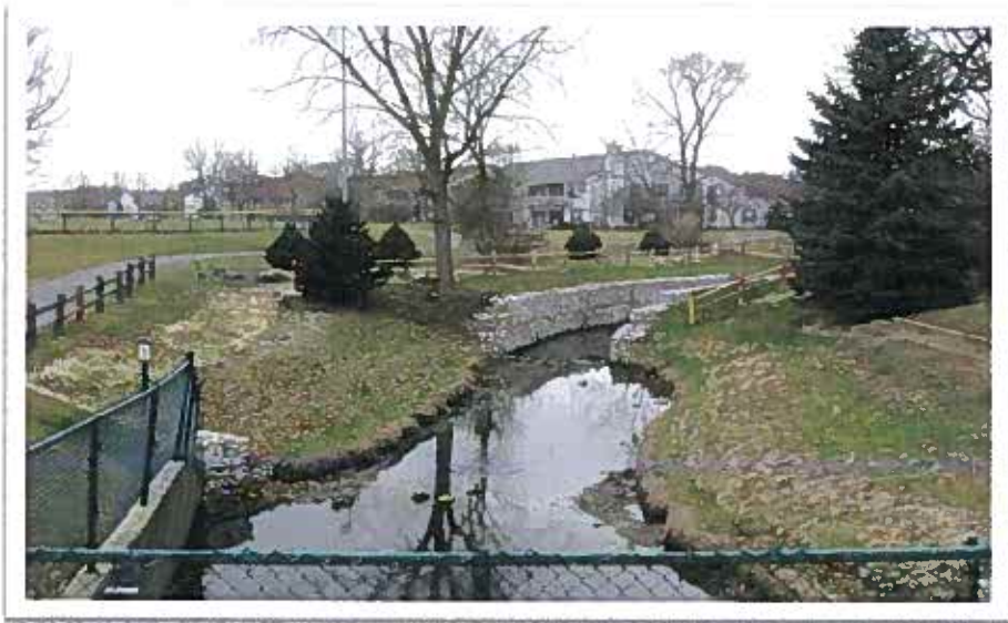
Looking downstream from Whispering Drive severe erosion at banks with poor vegetation (pre-construction). (Photo by M. Mann, Streamwood).
