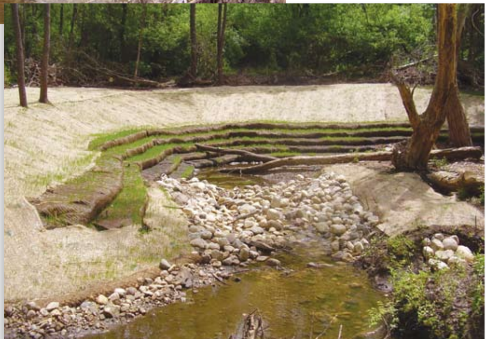
A section of severely eroded streambank before (top) and after (right) BMP construction. Stabilization practices include fiber roll with reshaped slope, rock riffle, and rock toe with vegetated geogrid, (photos courtesy of Ted Gray, Living Waters Consultants).
