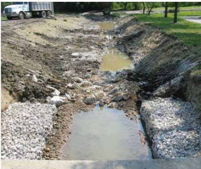
The same reach of White's Creek during (top) and after (bottom) BMP construction. Stabilization practices seen include bank regrading and vegetated buffer, gabion basket toe under vegetated geogrids, and rock riffles/pools (photos by H. Hudson, CMAP).
