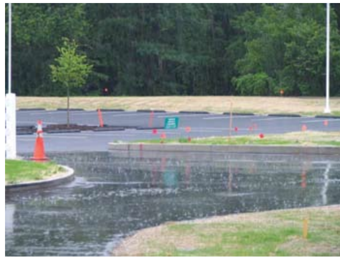
Rain falling on a conventional street surface (foreground) and generating stormwater runoff, a significant contributor to non point source pollution, next to a new porous-pavement parking lot (background) doing its job of preventing stormwater runoff that is typically associated with impervious surfaces (photo courtesy of Lake County Forest Preserves District).
