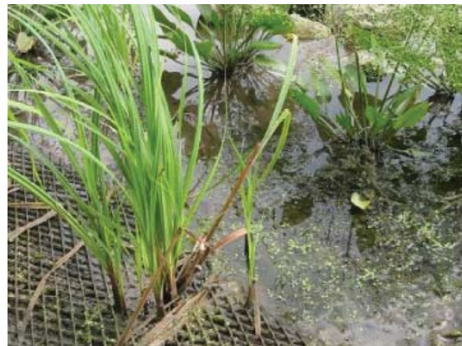
Common bur reed and water plantain, protected by a benthic mesh geoweb, are among the wetland plant species installed in the constructed planting shelf at Long Lake (photo by H. Hudson, CMAP).
