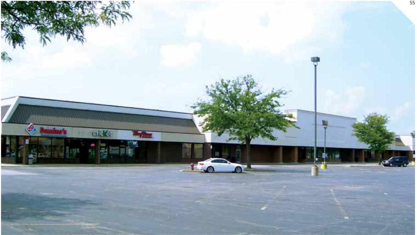
The redevelopment of some commercial facilities could include housing.
