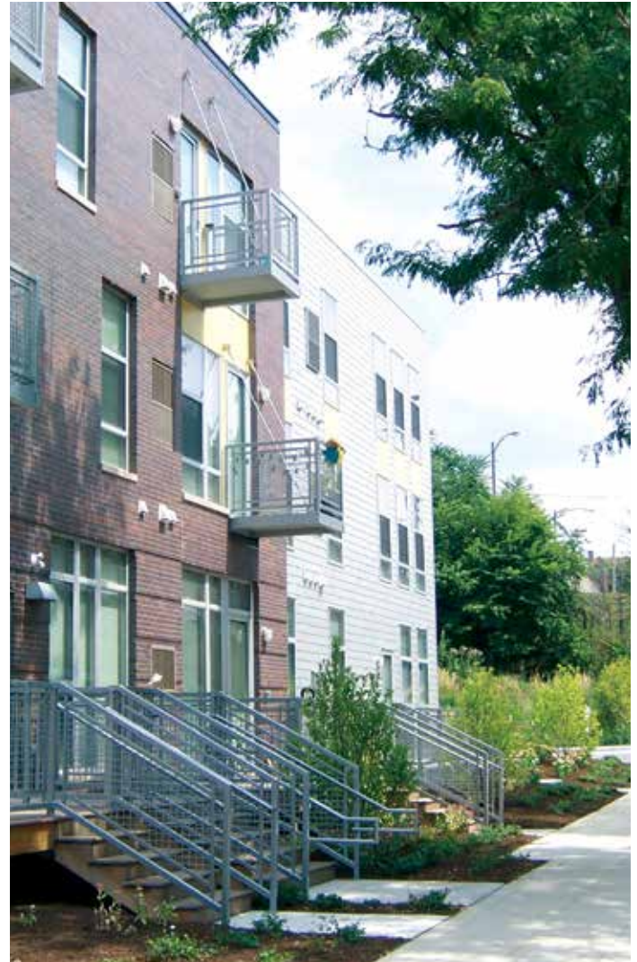
The Elgin Artspace Lofts include energy efficient features.
