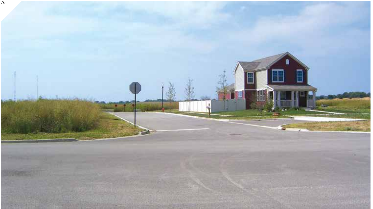
Unfinished or unbuilt single-family subdivisions in the western part of the City drive local capacity.
