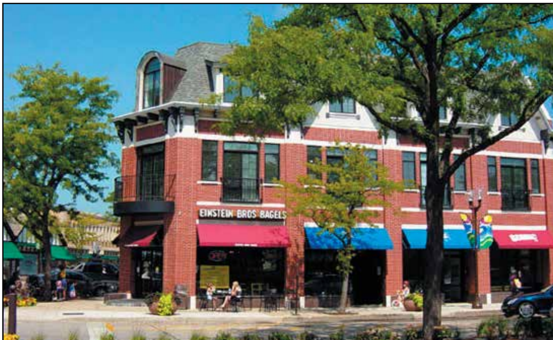
Example of mixed-use building on corner lot with articulated architecture.
