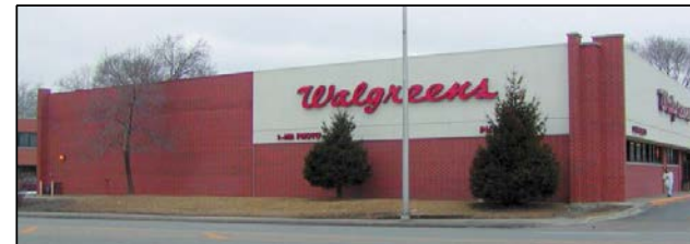
Inadequate fenestration blocks views of interior spaces. (4.7.4.7, 4.7.4.8, 4.7.4.9)
