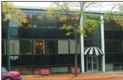
Building with no defined base, middle, or top. (4.7.2.1)
