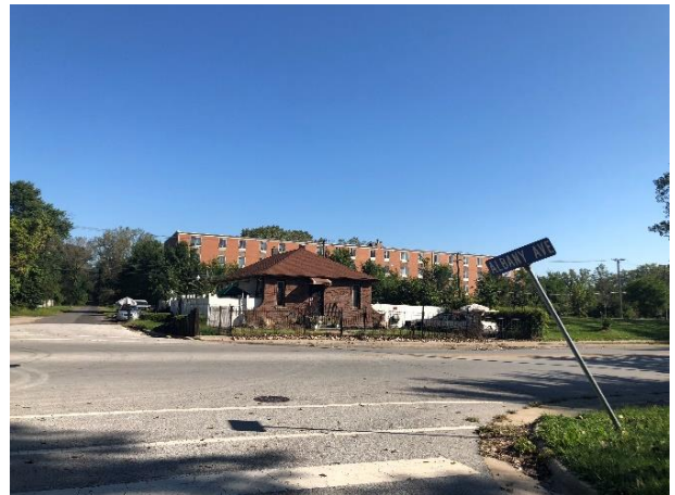
FIGURE 11: HOUSING STRUCTURE ON 139TH STREET JUST WEST OF METRA STATION
