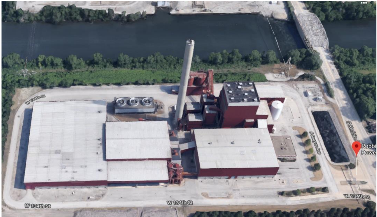
FIGURE 13: FORMER ROBBINS COMMUNITY POWER SITE
