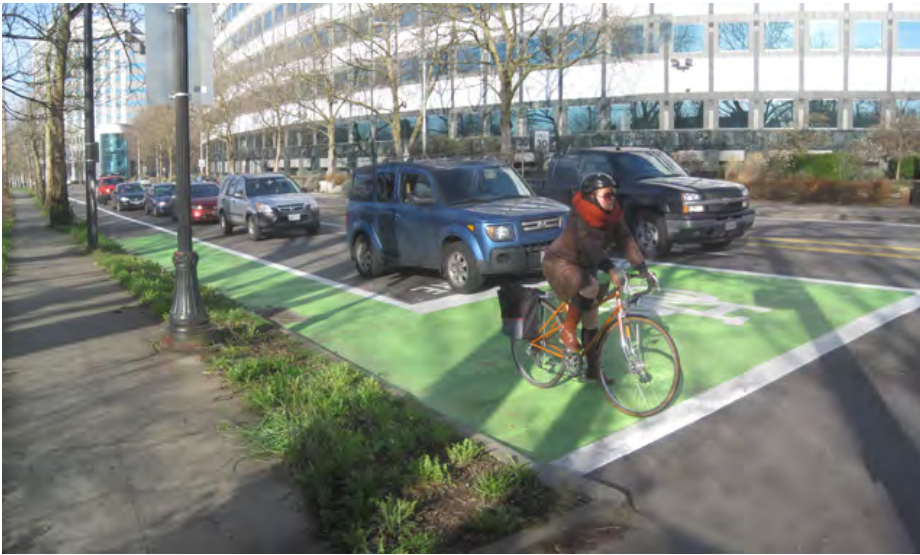
Figure 6: Installing bike boxes at intersections improve the visibility of bicyclists by providing them a space to wait in front of vehicles. Image credit: North American City Transportation Officials.
