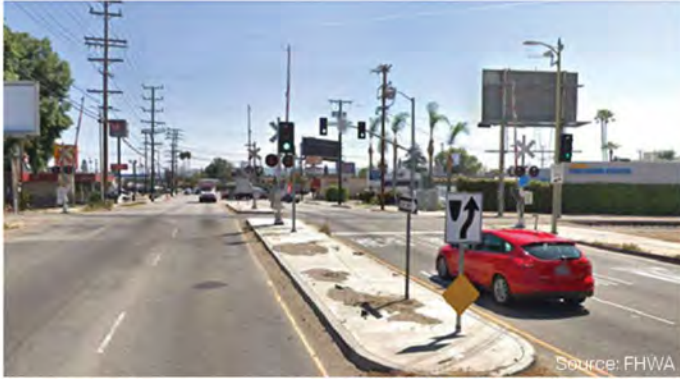
Concrete Median Barrier at Railroad Crossing
