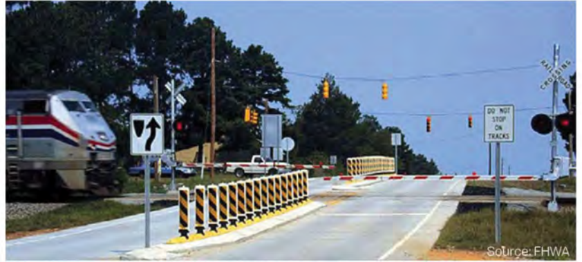
Mountable Raised Curb with Flexible Tubular Delineators
