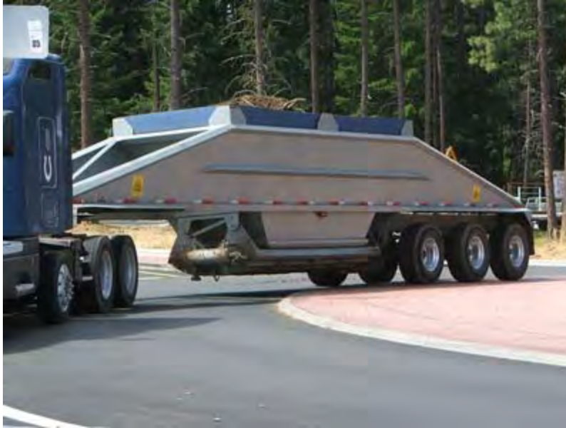
Figure 4: A truck apron in use. Image credits: Washington State DOT.
