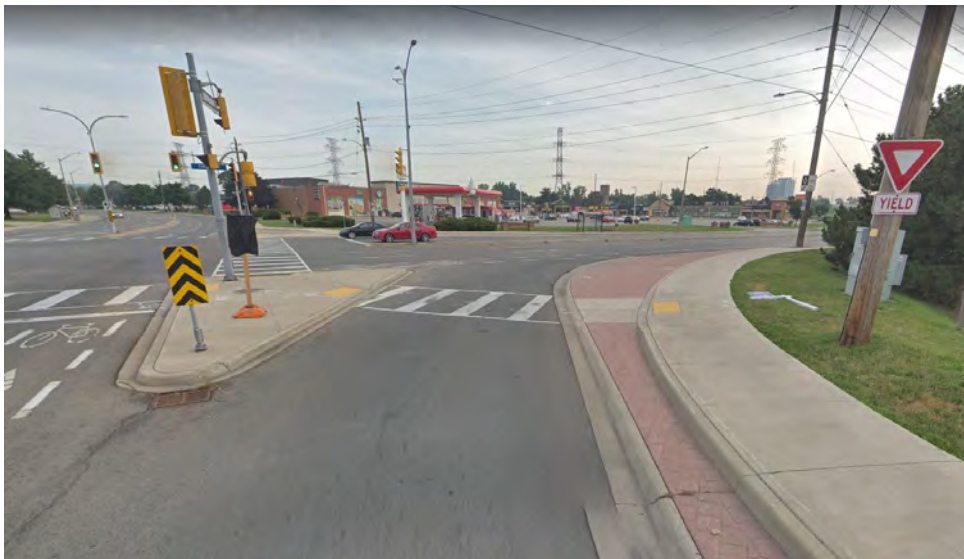
Figure 3: The red pavers indicate an example of a truck apron in Burlington, Ontario.. Image credits: Google Maps, 2018.
