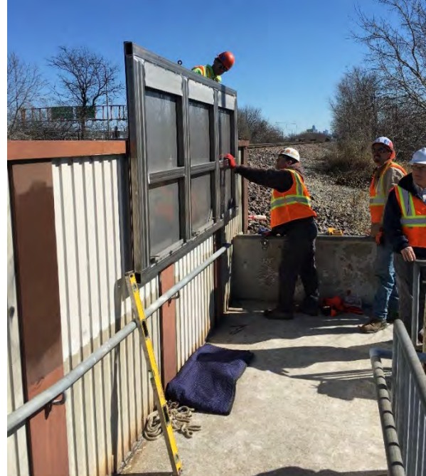
Installing the sign structure on the ramp to/from Metra
