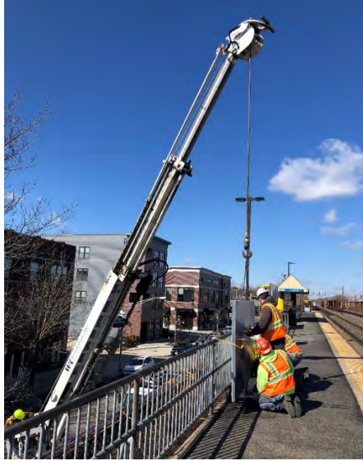
Lifting the sign structure to the Metra platform.
