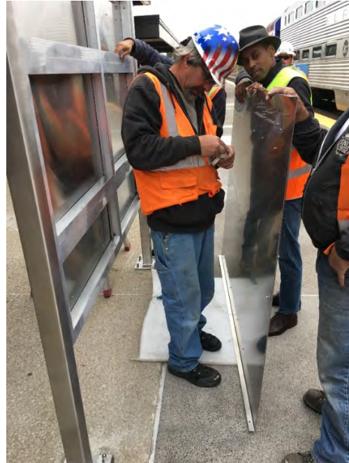
Installing the face plate on the sign structure
