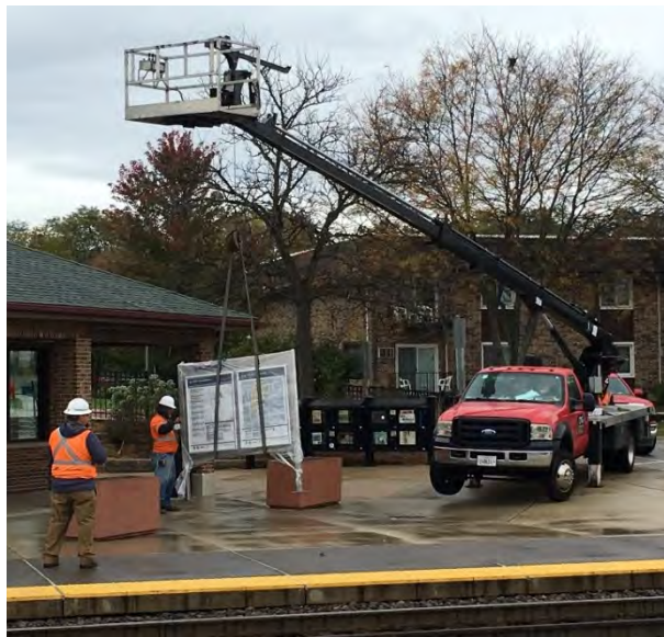
Lowering sign structure into place near the Metra station
