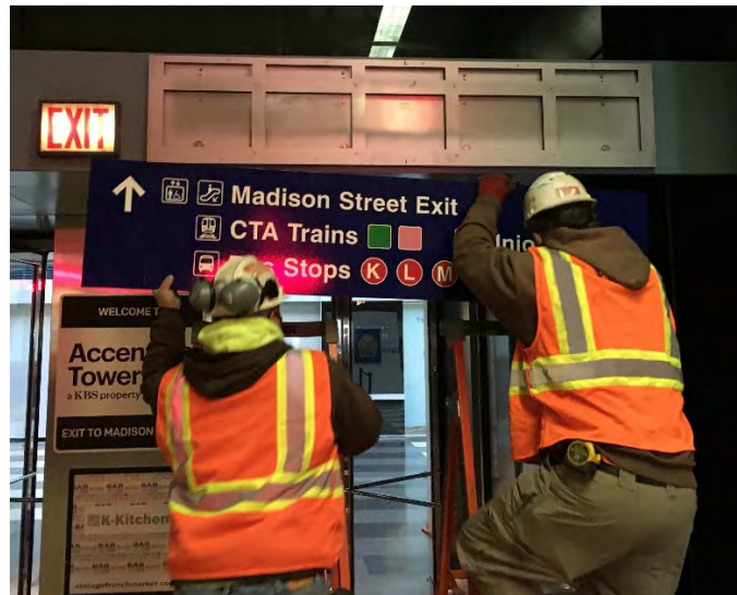
Installing sign over doors from platforms to Accenture Tower
