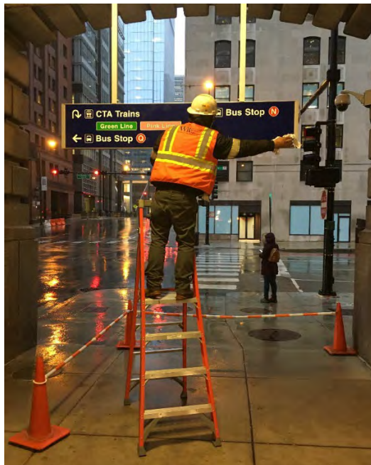
Installing sign above Washington St. sidewalk
