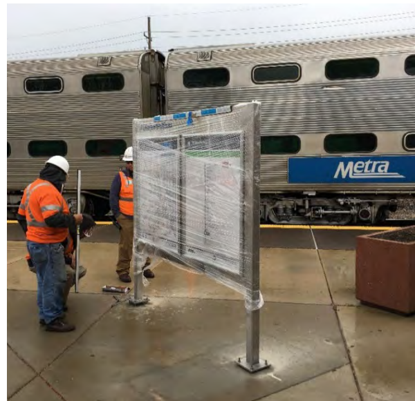
Mounting the sign structure to the concrete pavement
