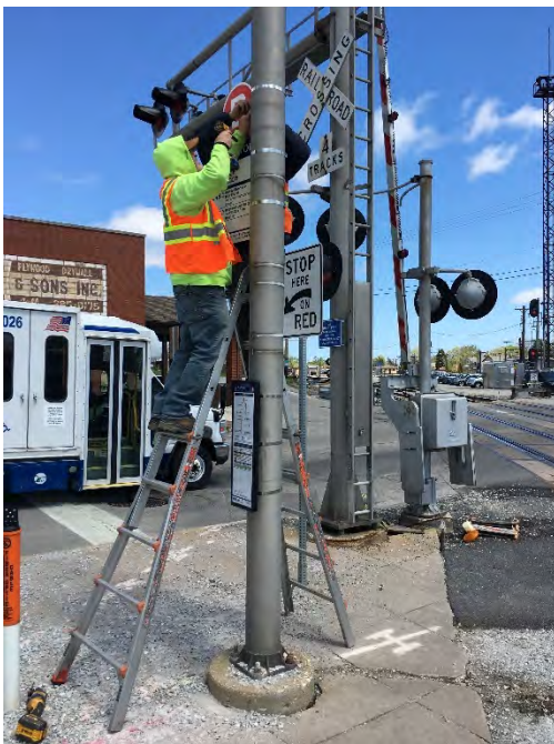
Installing bus stop sign near the grade crossing
