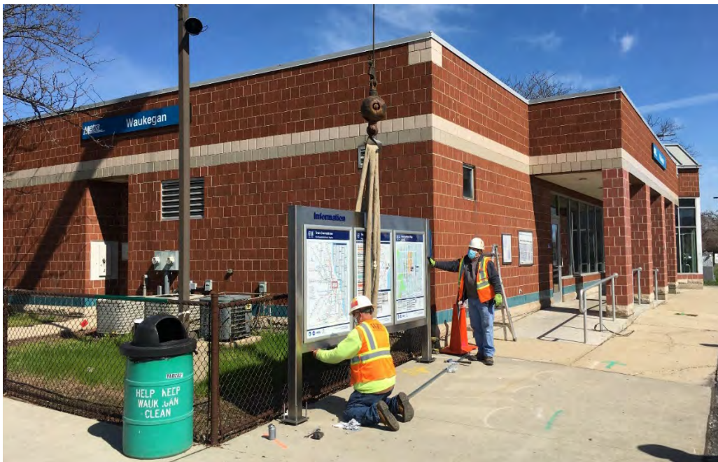
Installing the sign structure with maps near the Waukegan Metra station
